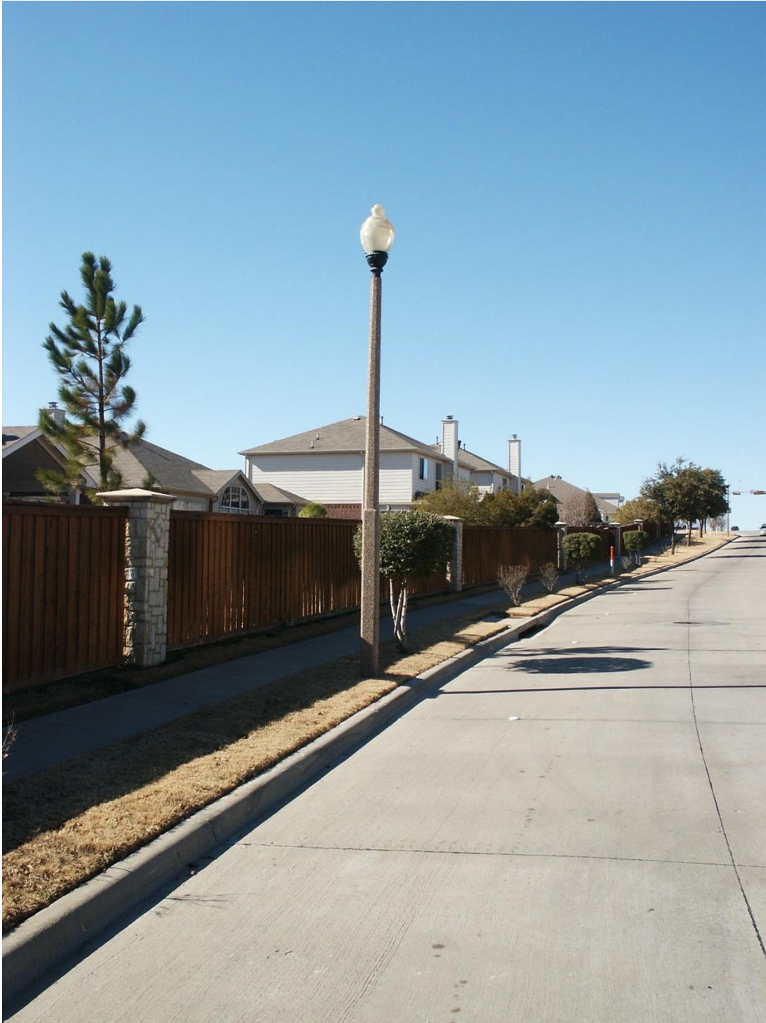
Typical 20 ft long (San Jacinto Brown finish) concrete streetlight pole (Exposed aggregate finish)
