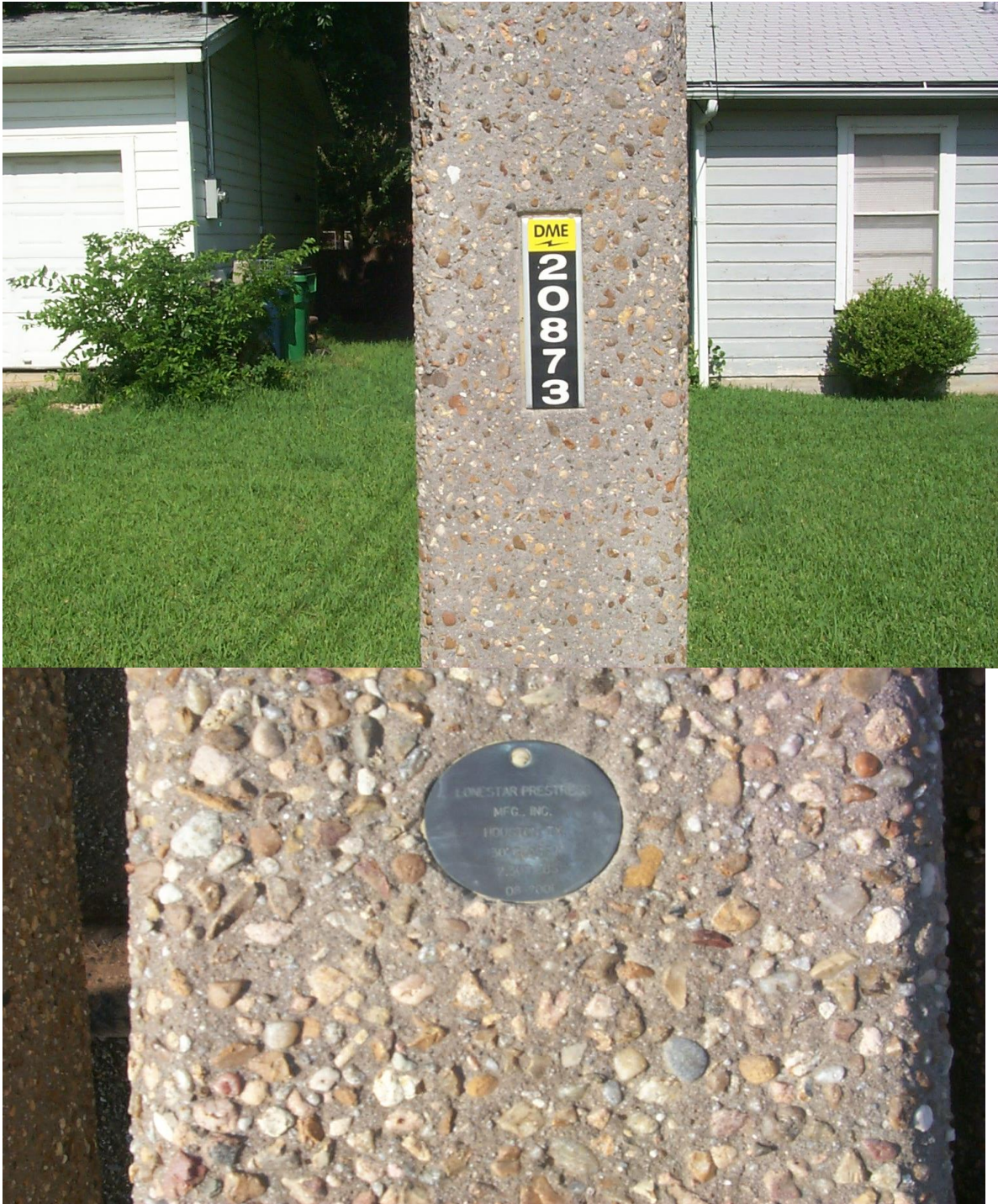
Close-up view of exposed aggregate surface on 20 foot pole and tag provisions
