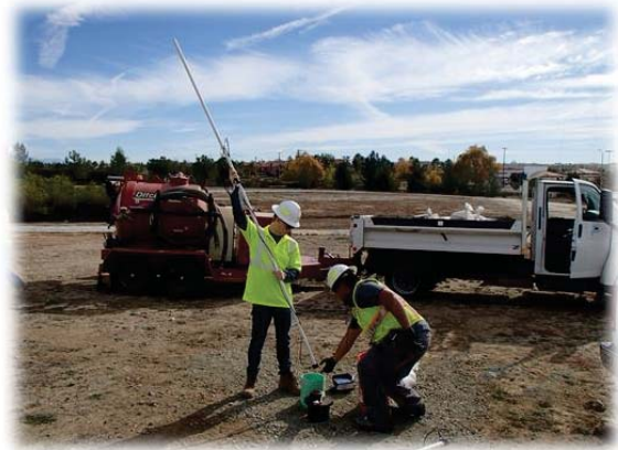
Figure 6. Tracking at a pothole location. Note the 8-inch green PVC sleeve and cap installed as part of the vacuum extraction excavation process.
