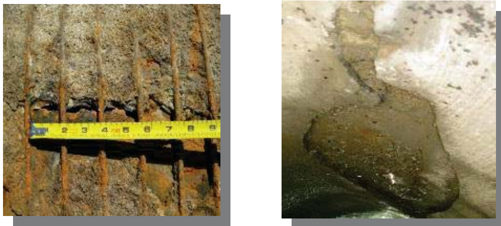
Figure 8: Examples of BWP deterioration: crack, extensive Corrosion, delamination and leakage
